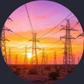
SENELEC – Senegal National Electricity Company 2017 – 2025 €10,783,000
